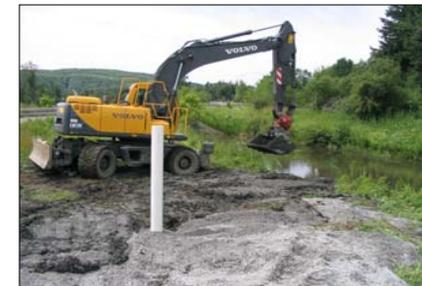
Water in streams, ponds and cisterns helps a fire department only when it is readily accessible and within close proximity of the fire. Installation of dry hydrants into strategically located water-bodies eliminates the inefficiency and complexity of long-distance water shuttle operations and also allows access to water sources directly from a roadway rather than traversing over soft or saturated ground.
